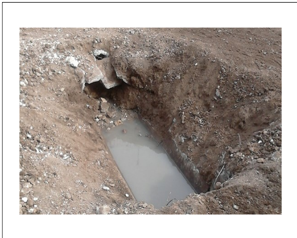
Illegal septic connection draining into storm water pipes leading to Port Vila Bay
