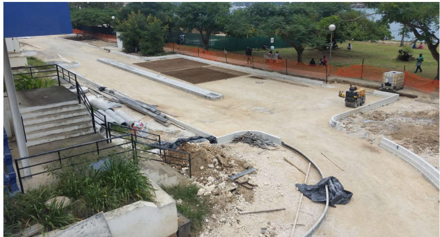
Construction works at George Kalsakau Drive after drains and kerbs were installed
