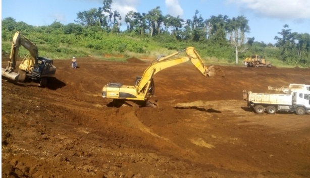
First lagoon under construction
