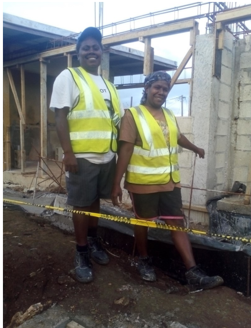
Serah Kalow (L) and Leikave Tom (R) pictured at the Seaside Tonga construction site
