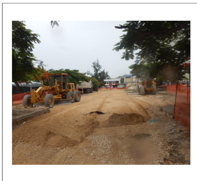
Start of construction works on George Kalsakau Drive March 2016
