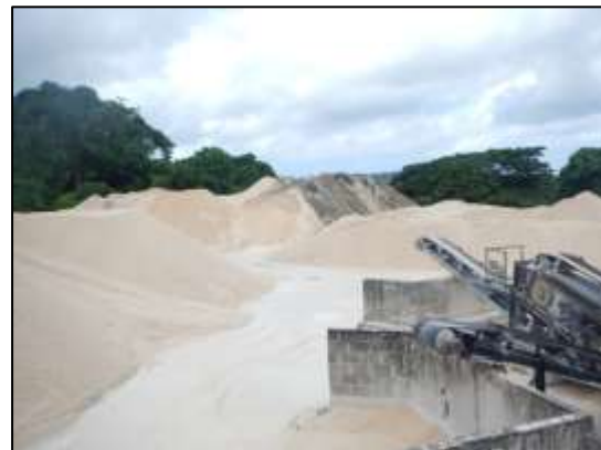
Plate 6 Aggregate processing plant at the quarry site
