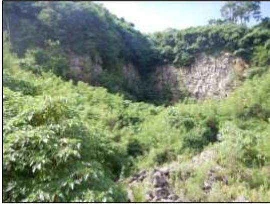
Plate 1 Existing quarry face
