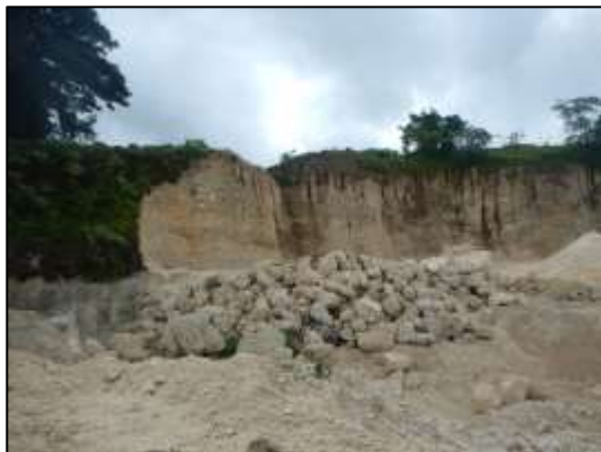
Plate 5 Existing quarry face and blasted material
