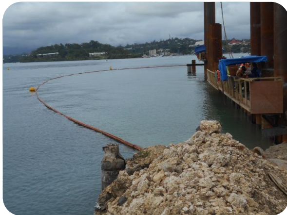
Silt Fence Installation
